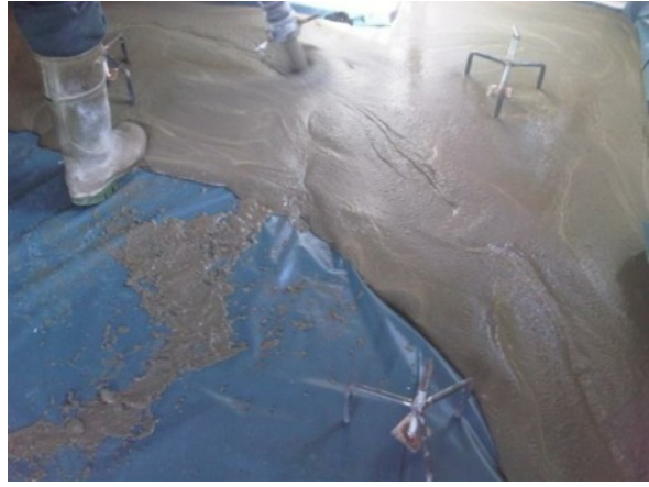
b. Screed being primed for levelling
