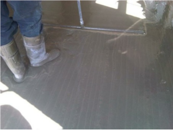
a. Screed being pumped
