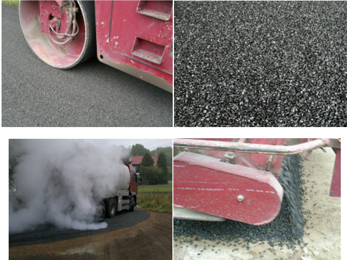
Figure 5.52 Hot Bitumen Chip and Spray.
