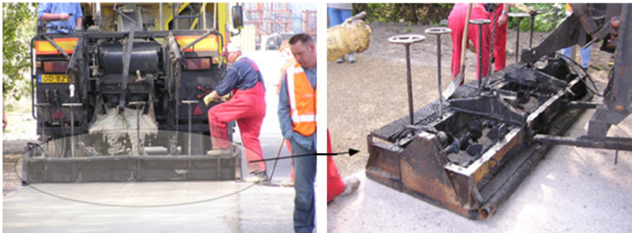
Figure 5.41 Placing of the ConcreCem Fine Aggregate(sand) Concrete.
