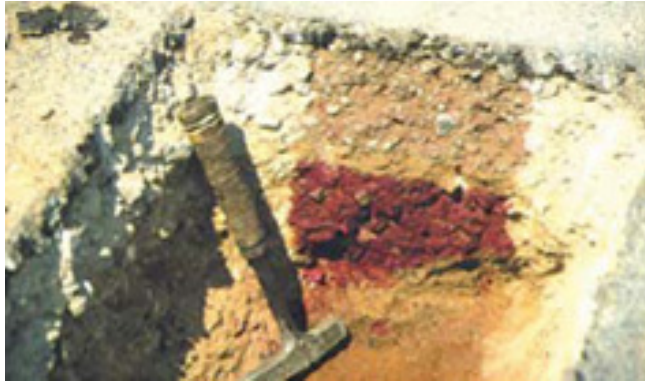
Figure 5.26 Phenolphthalein reaction in stabilised subbase.
