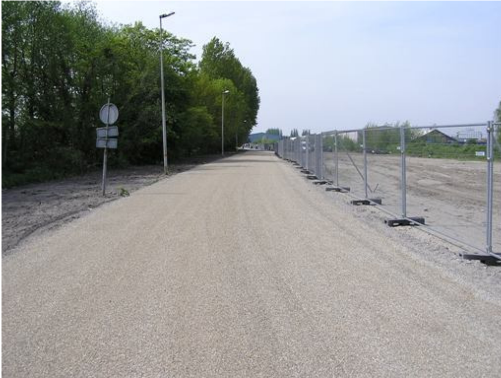
Figure 5.51 Finished single layer Chip and Spray.
