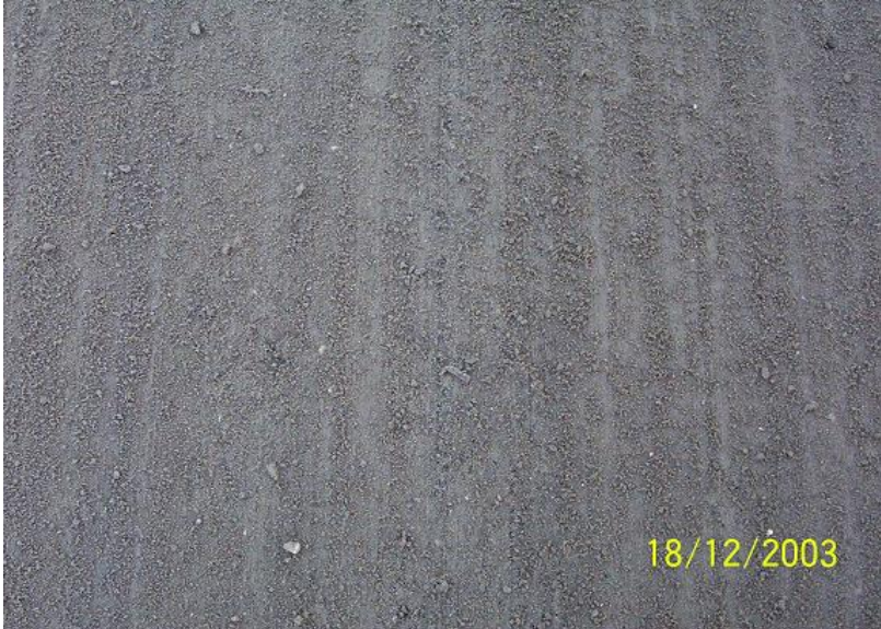
Figure 5.47 Mechanical Broom Finish.
