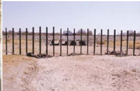
Figure 6.17 Vented drift.
