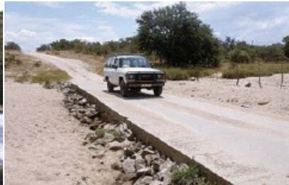
Figure 6.13 Vented drift.
