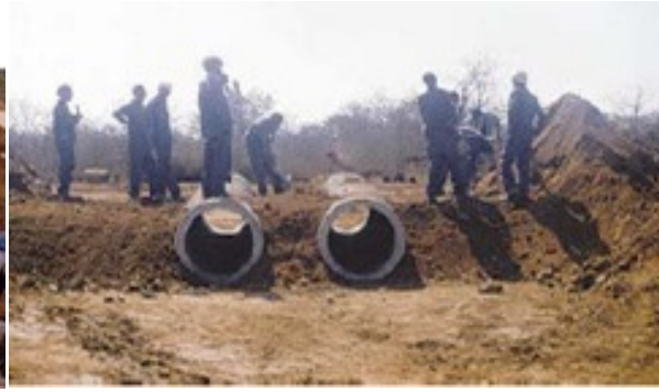
Figure 6.19 Vented drift.
