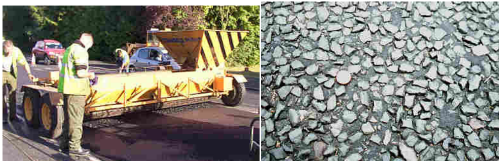
Figure 5.61 construction of asphalt
