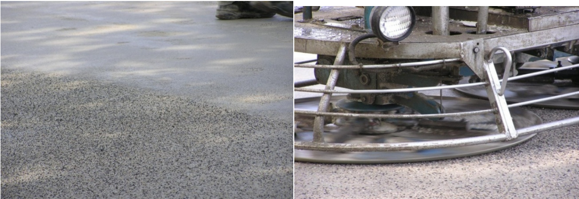
Figure 5.43 ConcreCem Fine Aggregate (sand) Concrete +Quartz Sand Finish.
