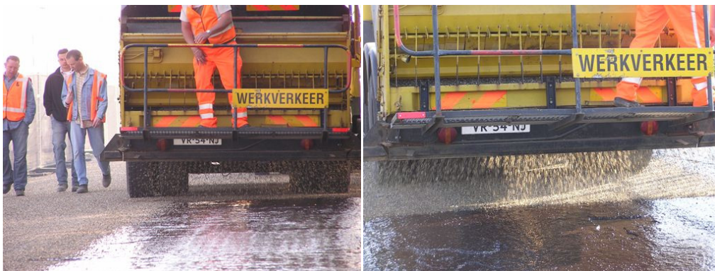
Figure 5.50 Applying chiped stone.
