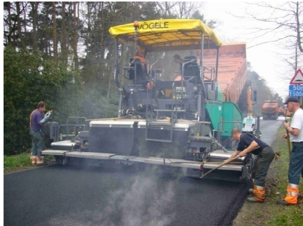
Figure 5.56 Applying asphalt layer.
