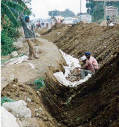
Figure 6.7 Construction of filler in drain.
