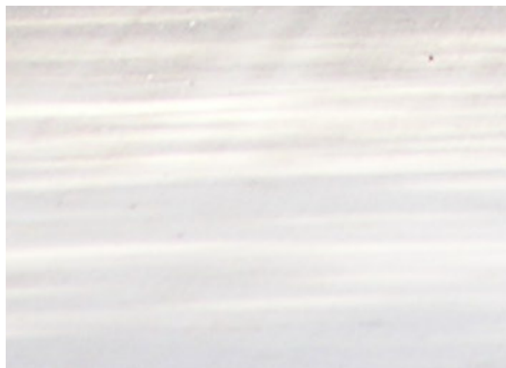
Figure 5.42 The look of the ConcreCem Fine Aggregate(sand) Concrete Finish.
