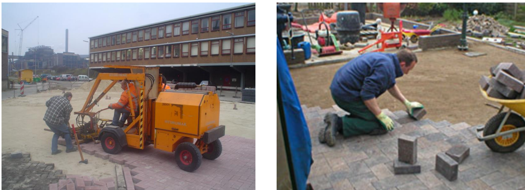
Figure 5.55 Applying paving bricks (automatically or manually).
