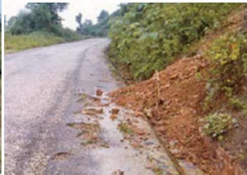
Figure 6.2 Damaged drainage.
