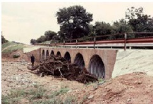
Figure 6.14 Inadequate culvert.
