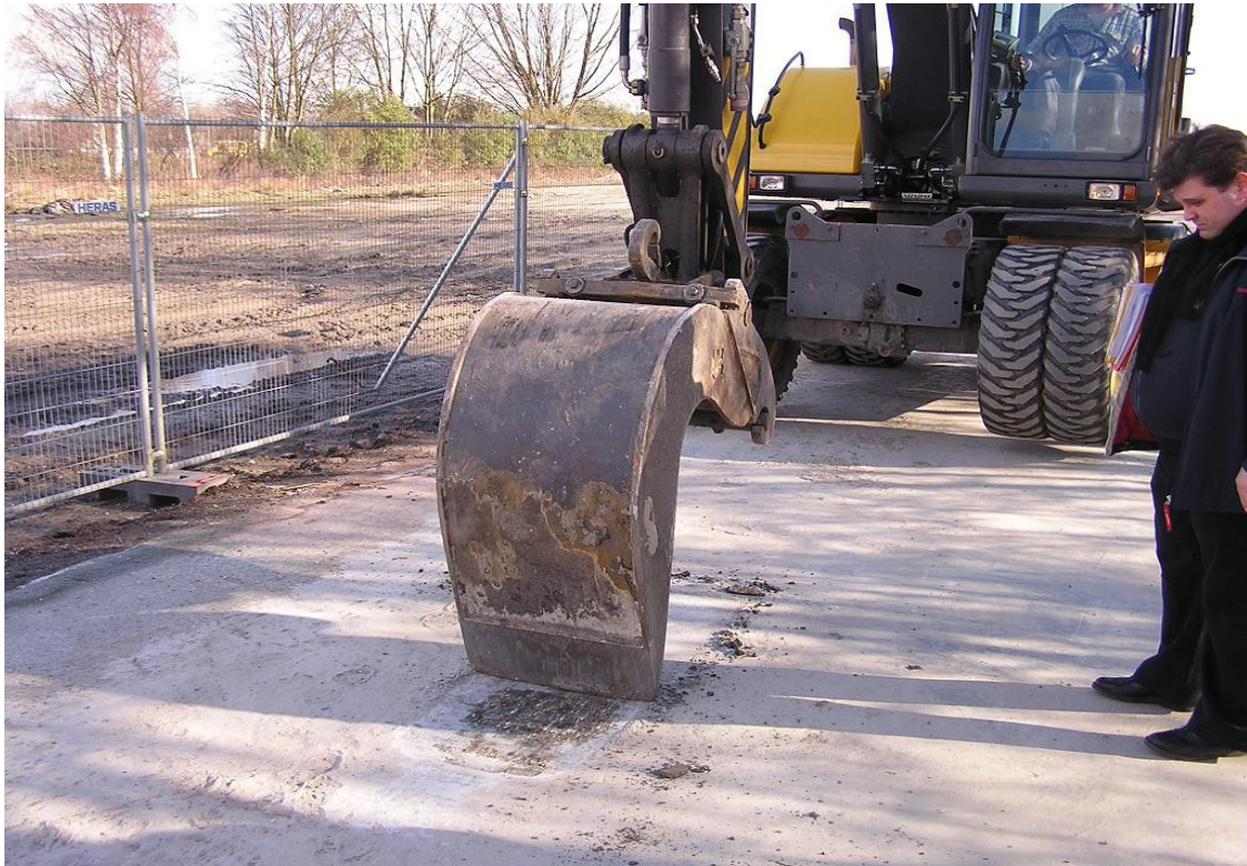
Figure 5.54 Gravel+RoadCem/Cement Slurry Finish
