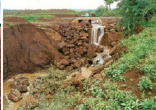
Figure 6.21 Vented drift.
