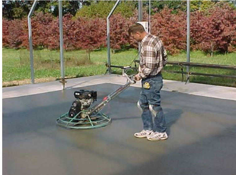
Figure 5.44 Implementing Smooth finisher.
