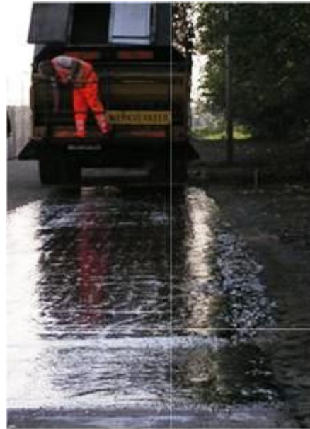
Figure 5.49 Cold Aqueous Bitumen Priming.
