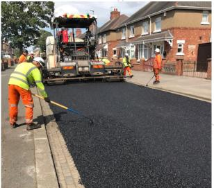
Testing confirmed the characteristic poor foundation and tar contamination. LWD's were converted to an underlying 2-4% CBR value. The challenge around the foundation issues led SPL to propose the inclusion of RoadCem.
