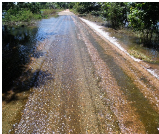
Figure 1.1: Road construction based on the PowerCem Technology
